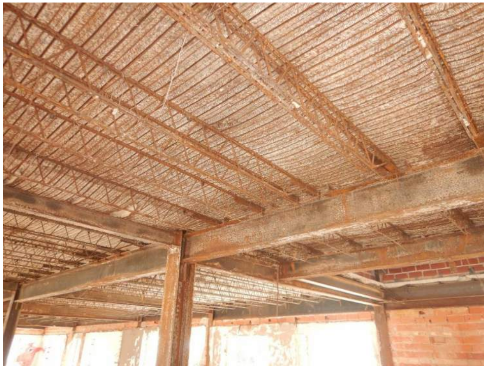
Photo 2: Detail of Berloy Ribplex from demo material pile
