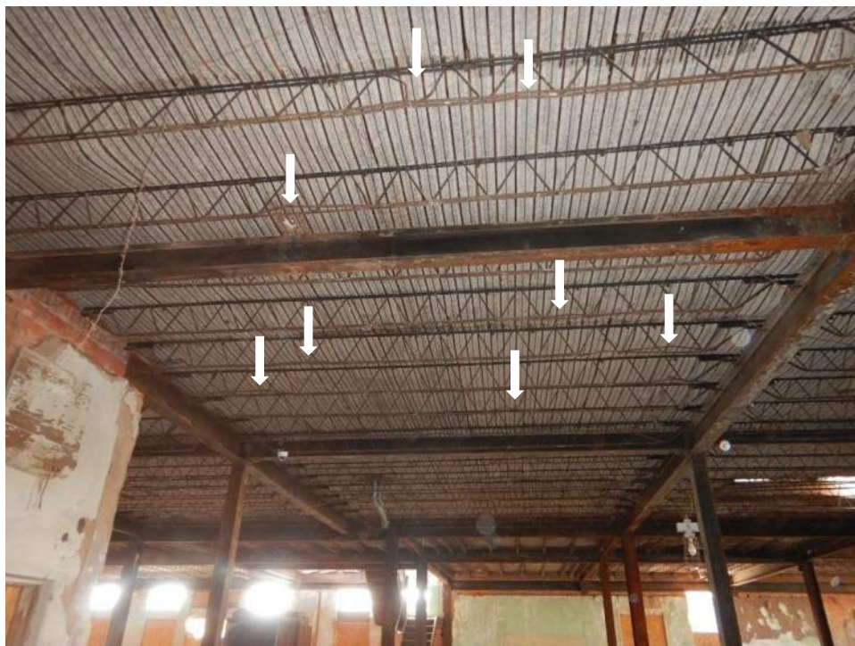
Photo 12: Example of Damaged Steel Joists in a 2 nd Level Bay
