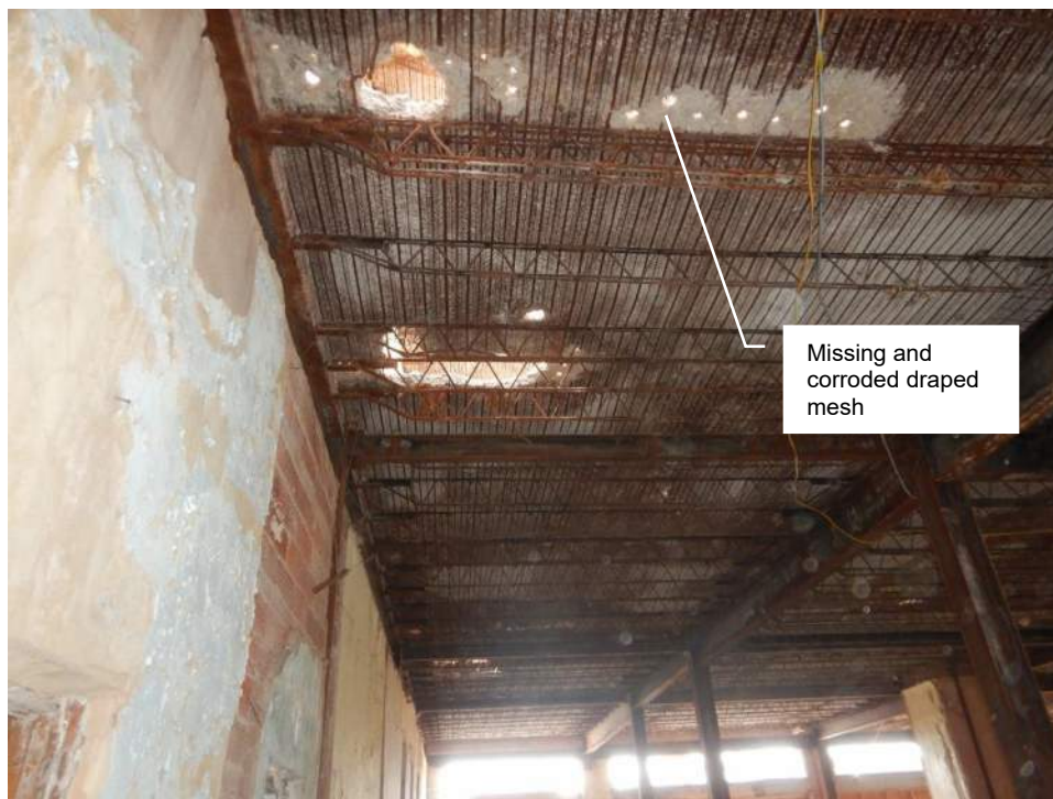
Photo 6: Corroded Joist Bearing and Beam Corrosion
