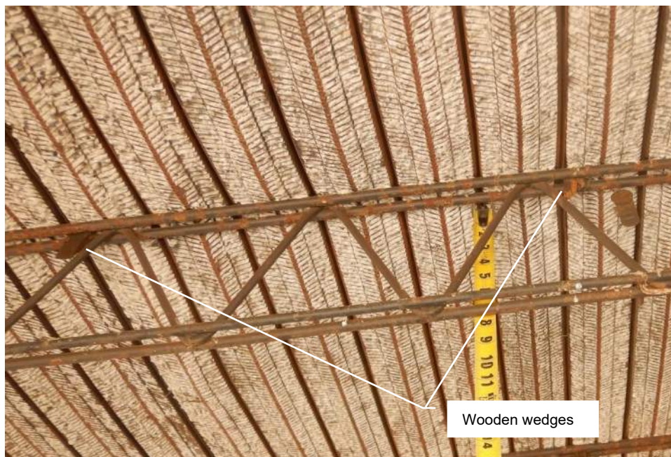
Photo 10: Concrete Fill over Berloy Ribplex
