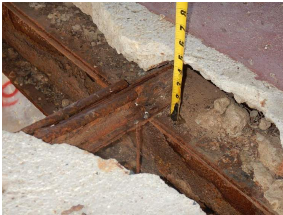
Photo 6: Corroded Joist Bearing and Beam Corrosion
