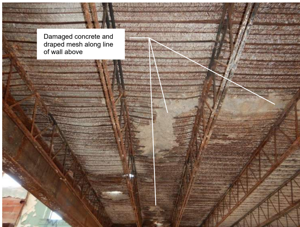
Photo 12: Example of Damaged Steel Joists in a 2 nd Level Bay
