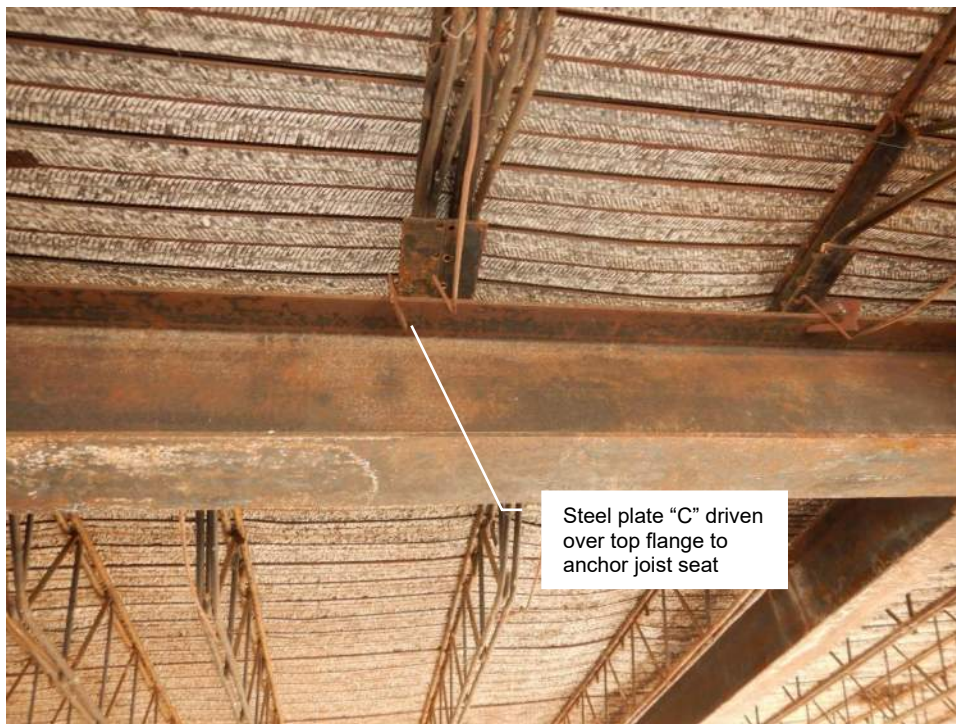
Photo 8: Typical Joist Connection to Steel Beams
