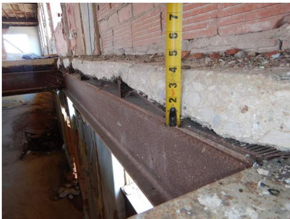
Photo 10: Concrete Fill over Berloy Ribplex
