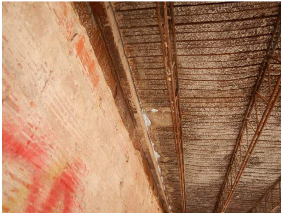
Photo 8: Typical Joist Connection to Steel Beams
