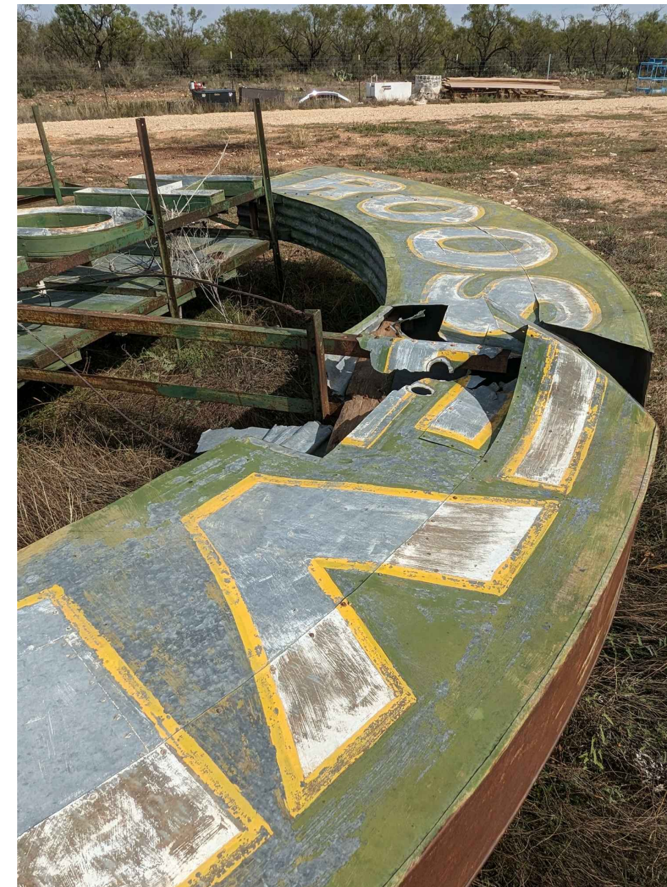
PHOTO EXISTING SIGN CONDITION N.T.S.
