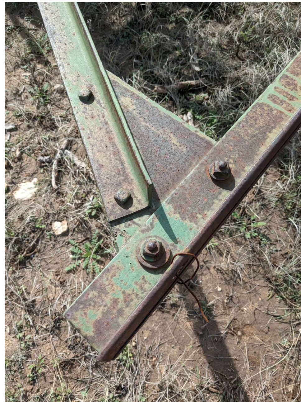
PHOTO EXISTING SIGN CONDITION N.T.S.
