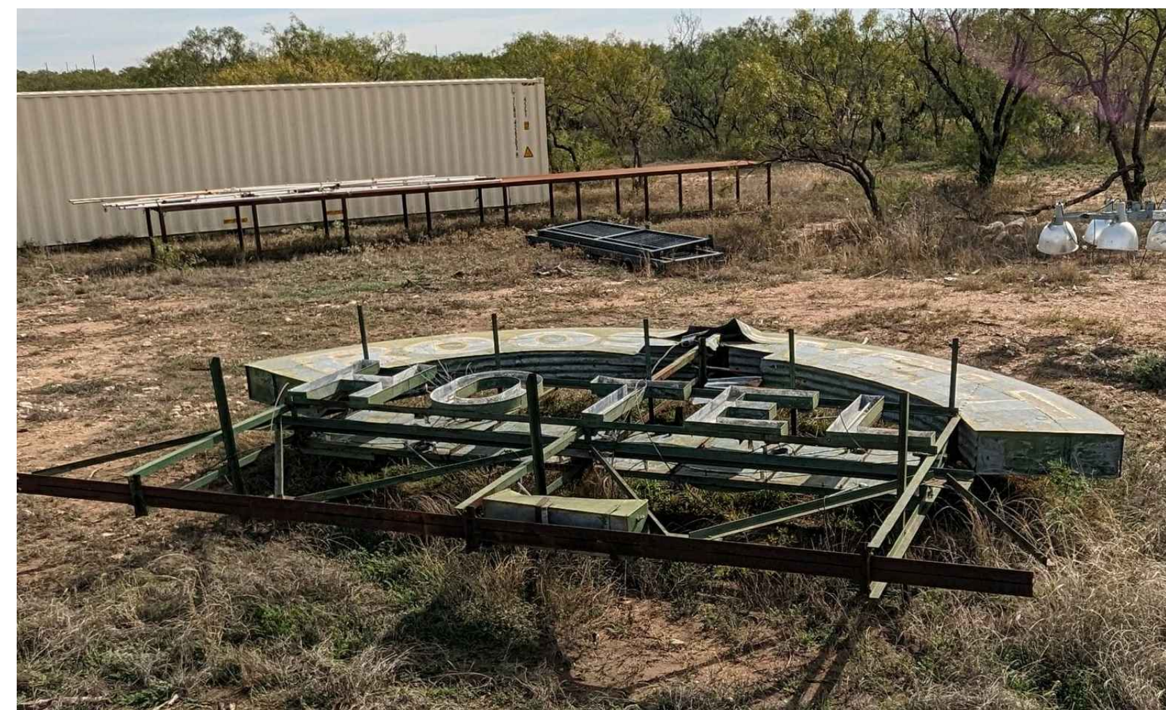
PHOTO EXISTING SIGN CONDITION N.T.S.
