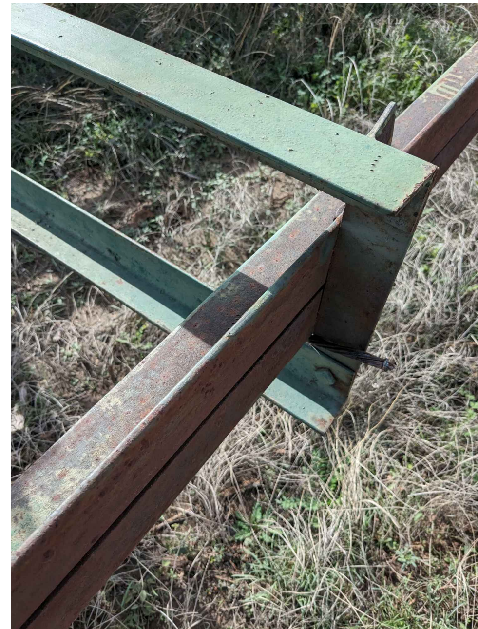
PHOTO EXISTING SIGN CONDITION N.T.S.
