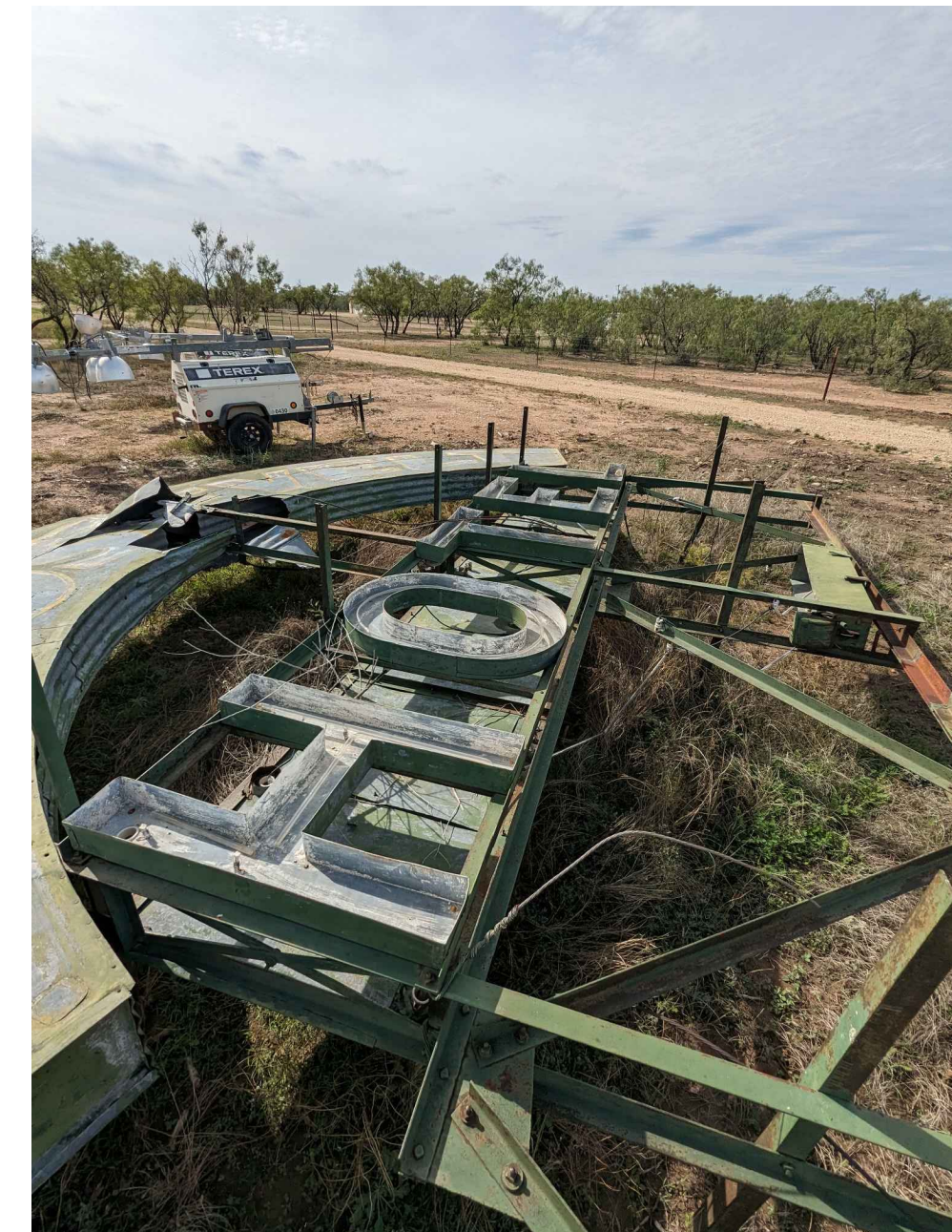
PHOTO EXISTING SIGN CONDITION N.T.S.
