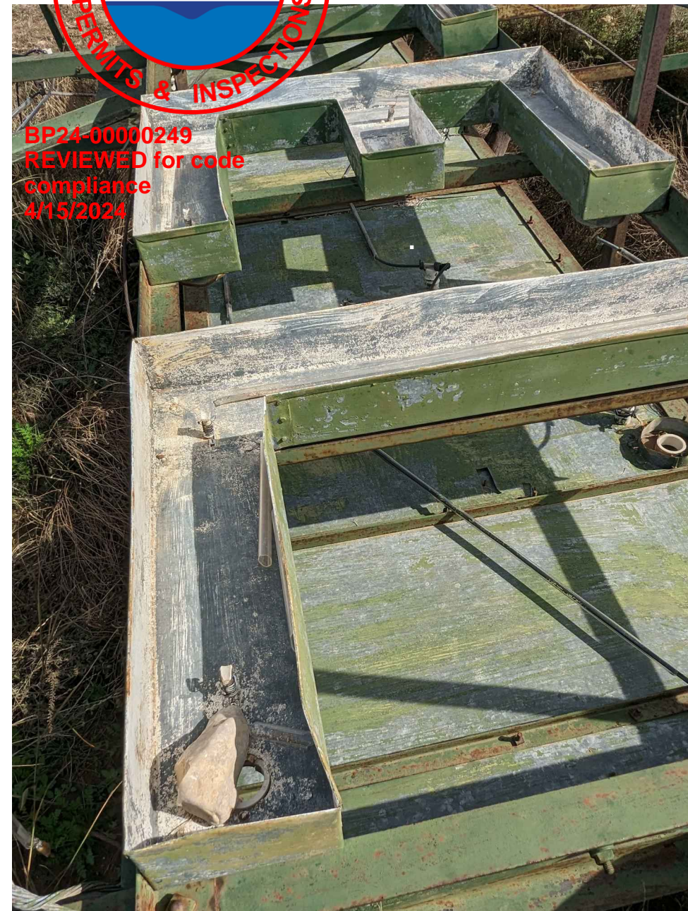
PHOTO EXISTING SIGN CONDITION N.T.S.
