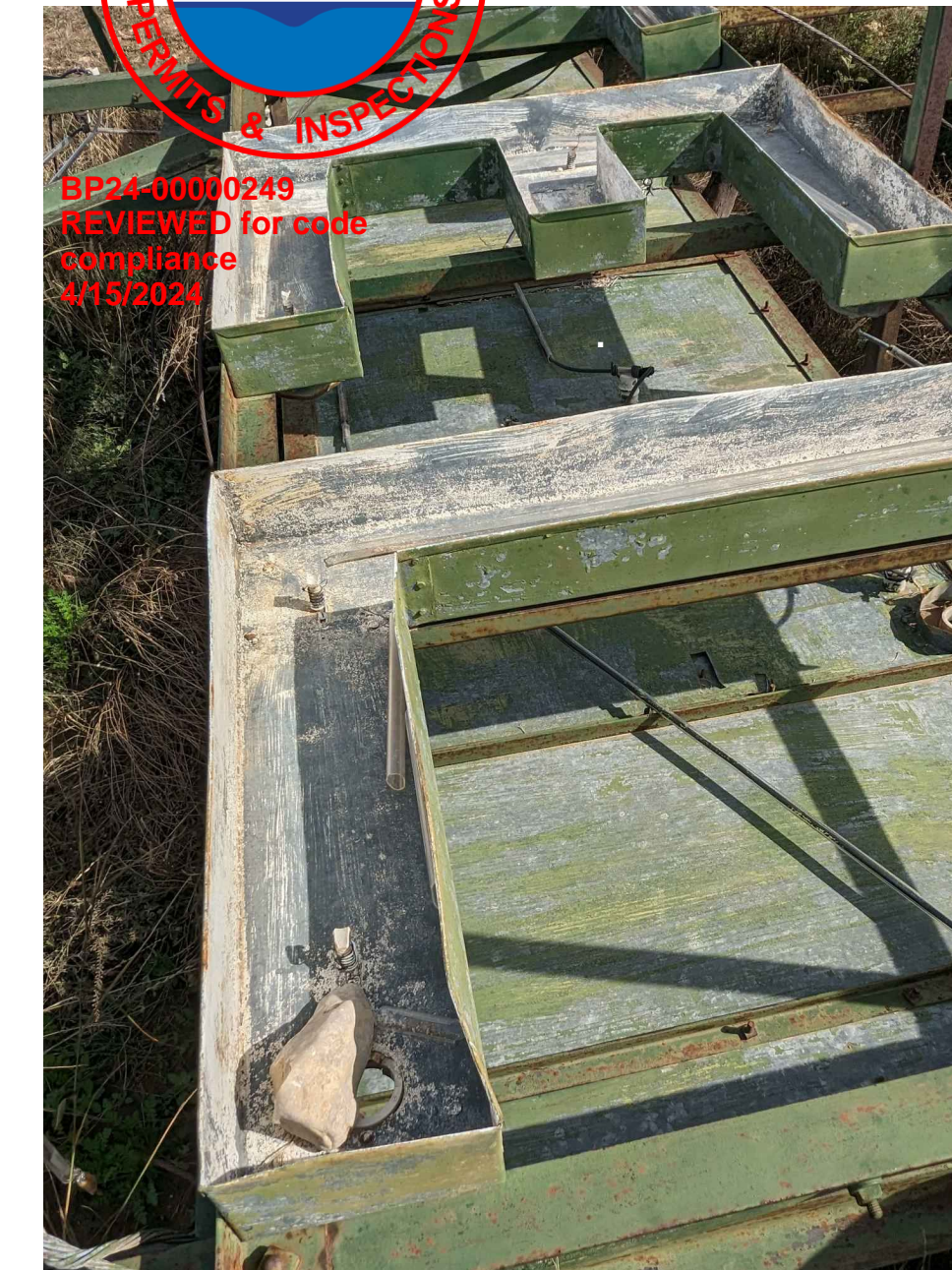
PHOTO EXISTING SIGN CONDITION N.T.S.
