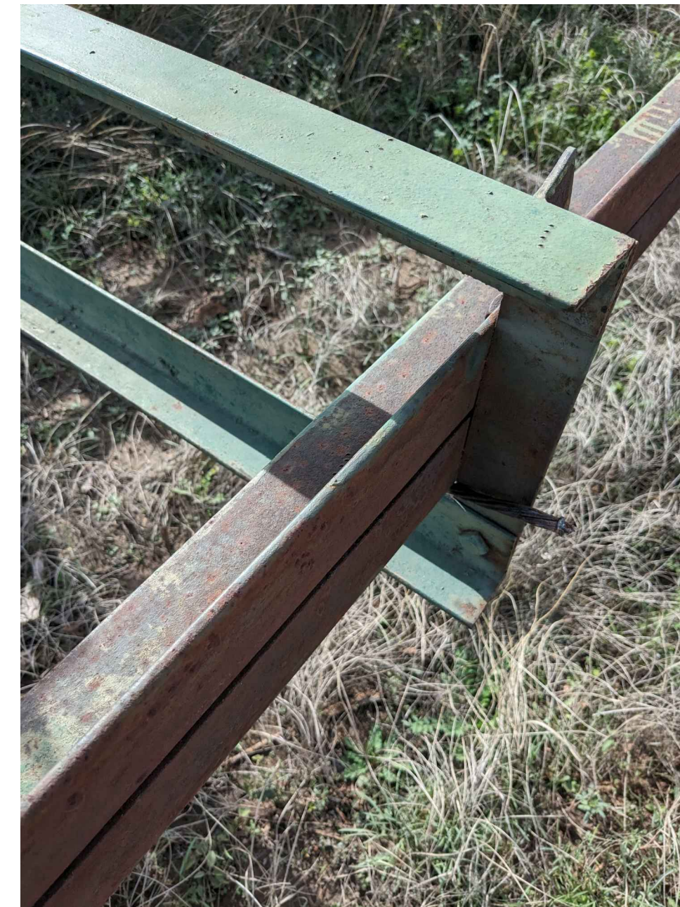
PHOTO EXISTING SIGN CONDITION N.T.S.
