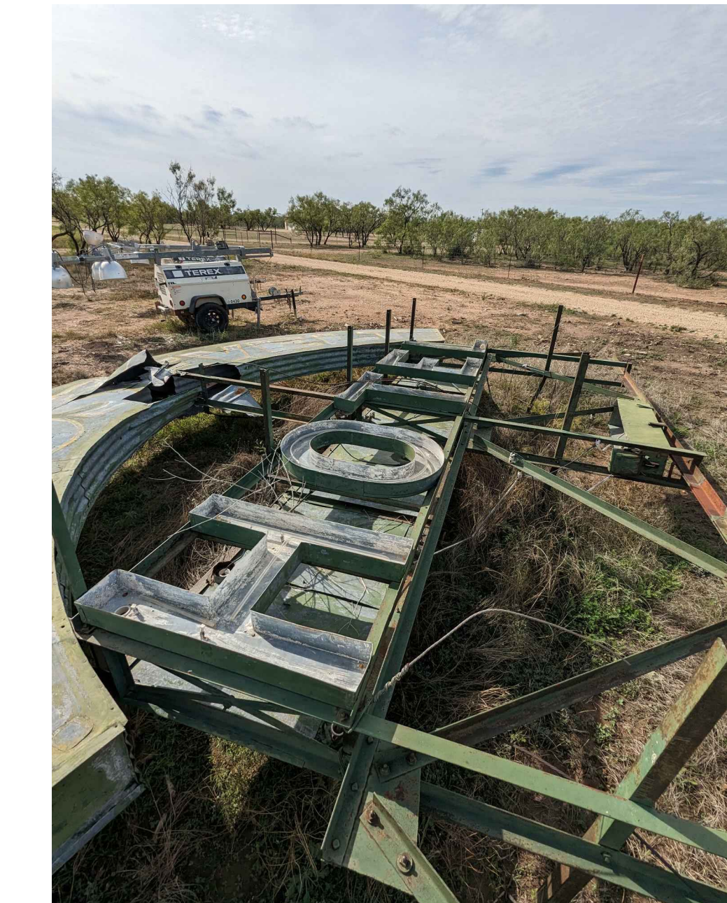
PHOTO EXISTING SIGN CONDITION N.T.S.
