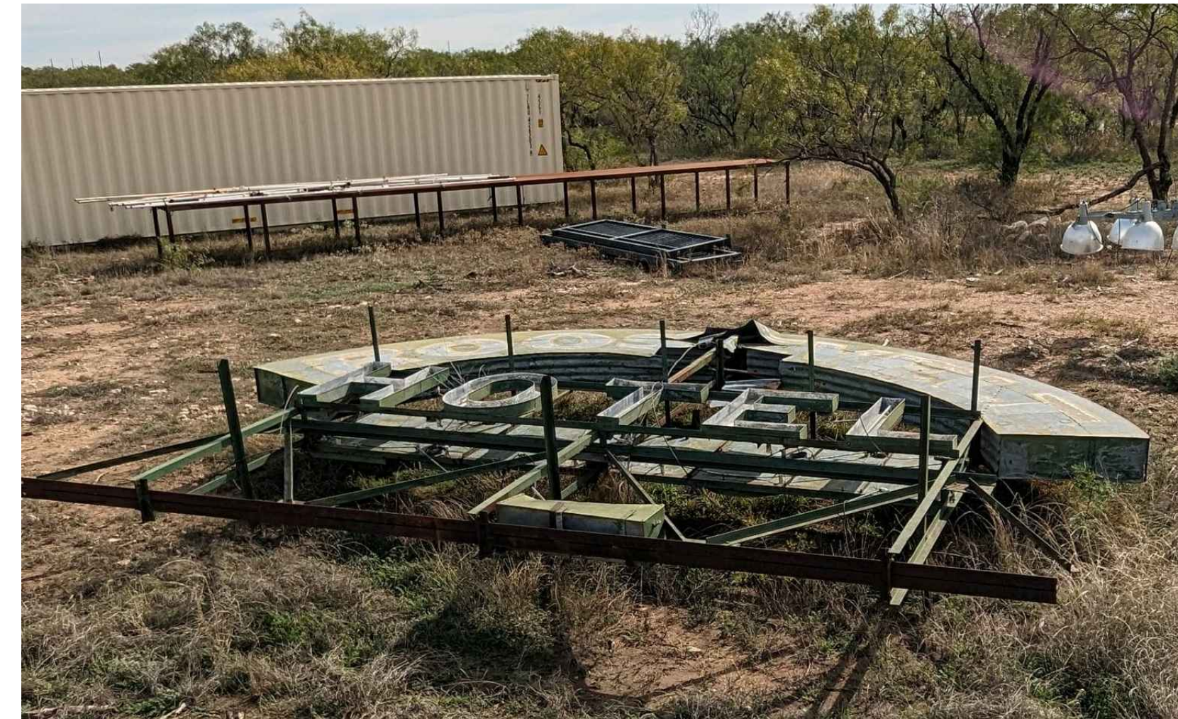
PHOTO EXISTING SIGN CONDITION N.T.S.
