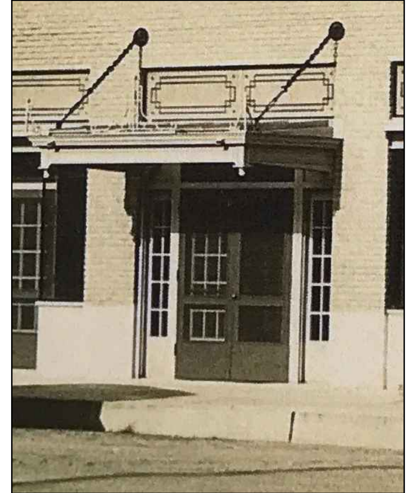
N. CHADBORNE STREET (DR #101) HISTORIC ENTRANCE PHOTOGRAPH NO SCALE
