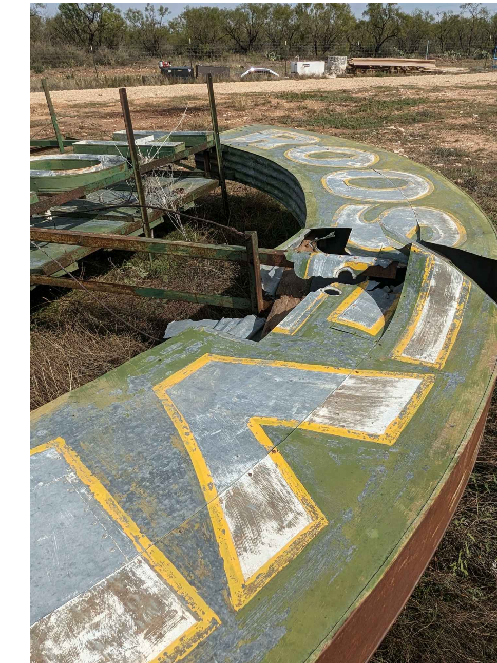
PHOTO EXISTING SIGN CONDITION N.T.S.
