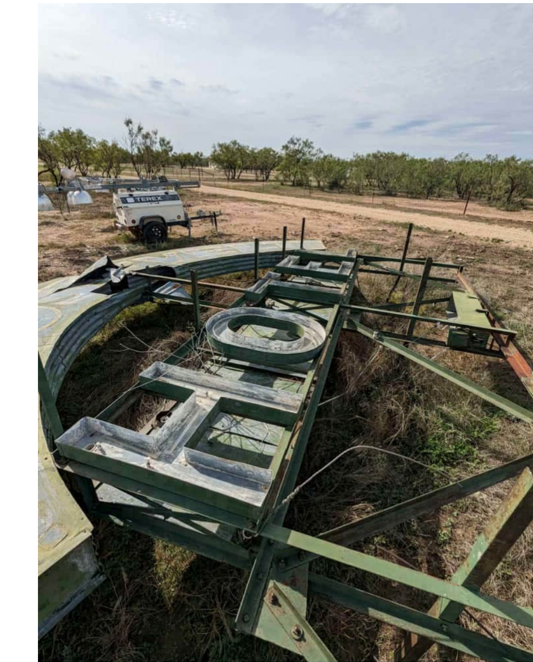
PHOTO EXISTING SIGN CONDITION N.T.S.
