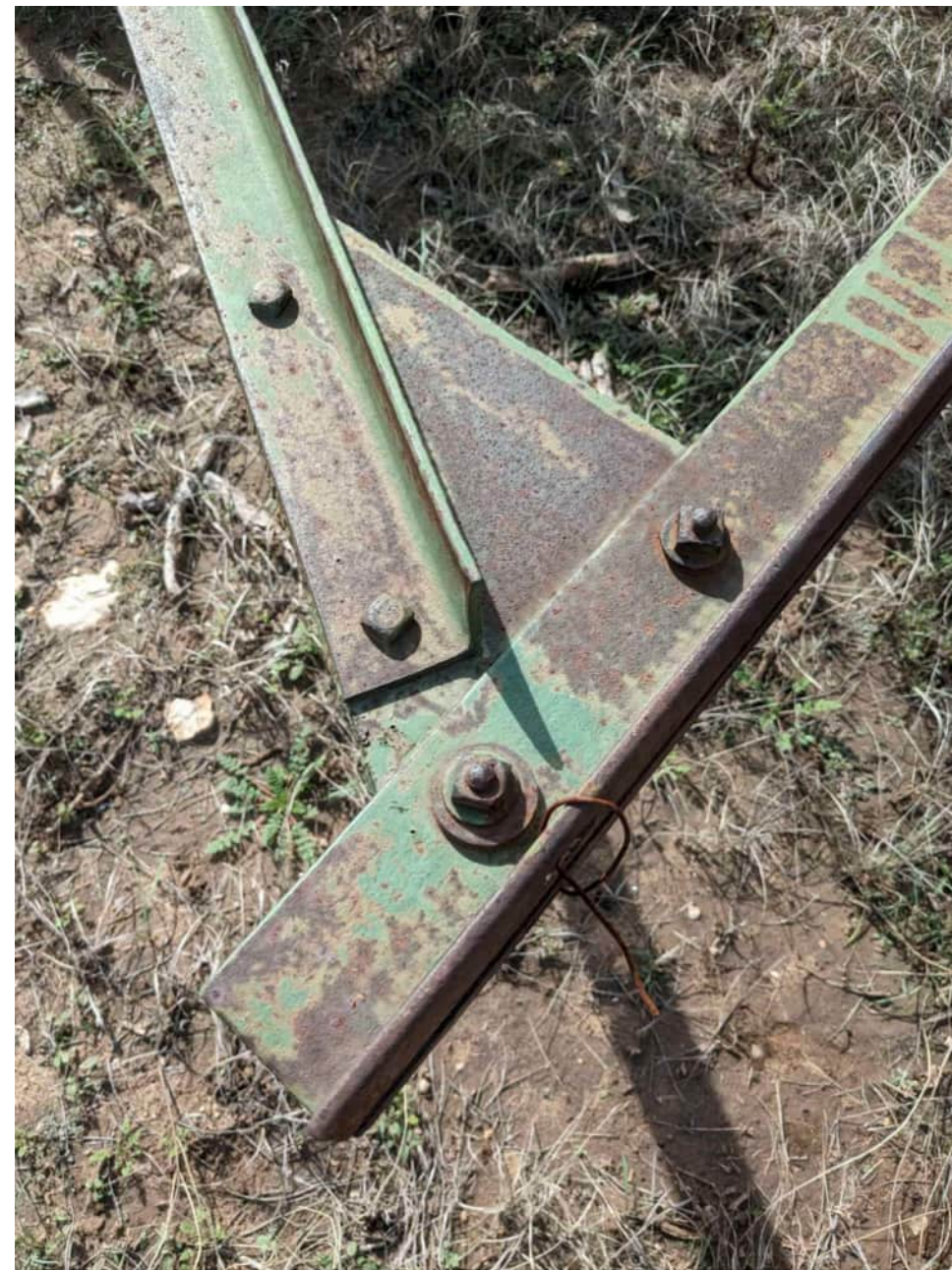
PHOTO EXISTING SIGN CONDITION N.T.S.
