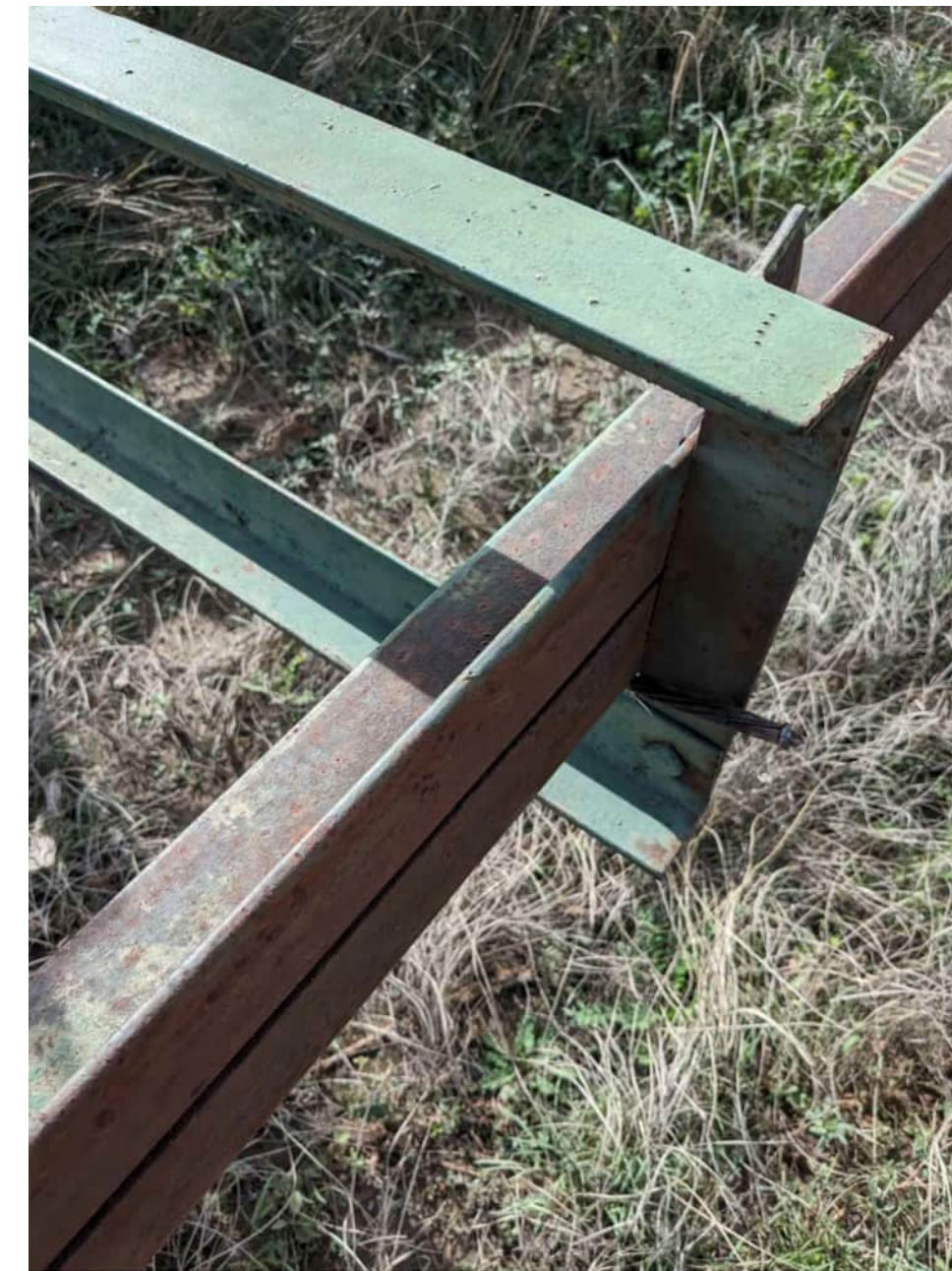
PHOTO EXISTING SIGN CONDITION N.T.S.
