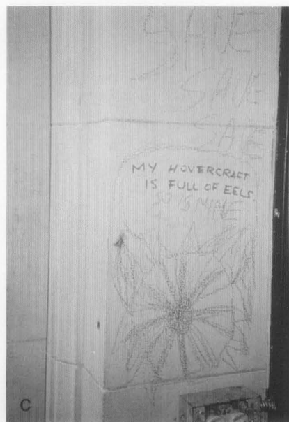
Figure 3 (a-d). A wide variety of materials is used to make surface-applied graffiti on masonry, including (a) chalk, (b) felt-tip marker, (c) felt-tip marker combined with crayon, and (d) felt-tip marker and spray paint on concrete. Photos: (a) Anne Grimmer, (b) Frances Gale, (c) Martin Weaver, (d) Anne Grimmer.
