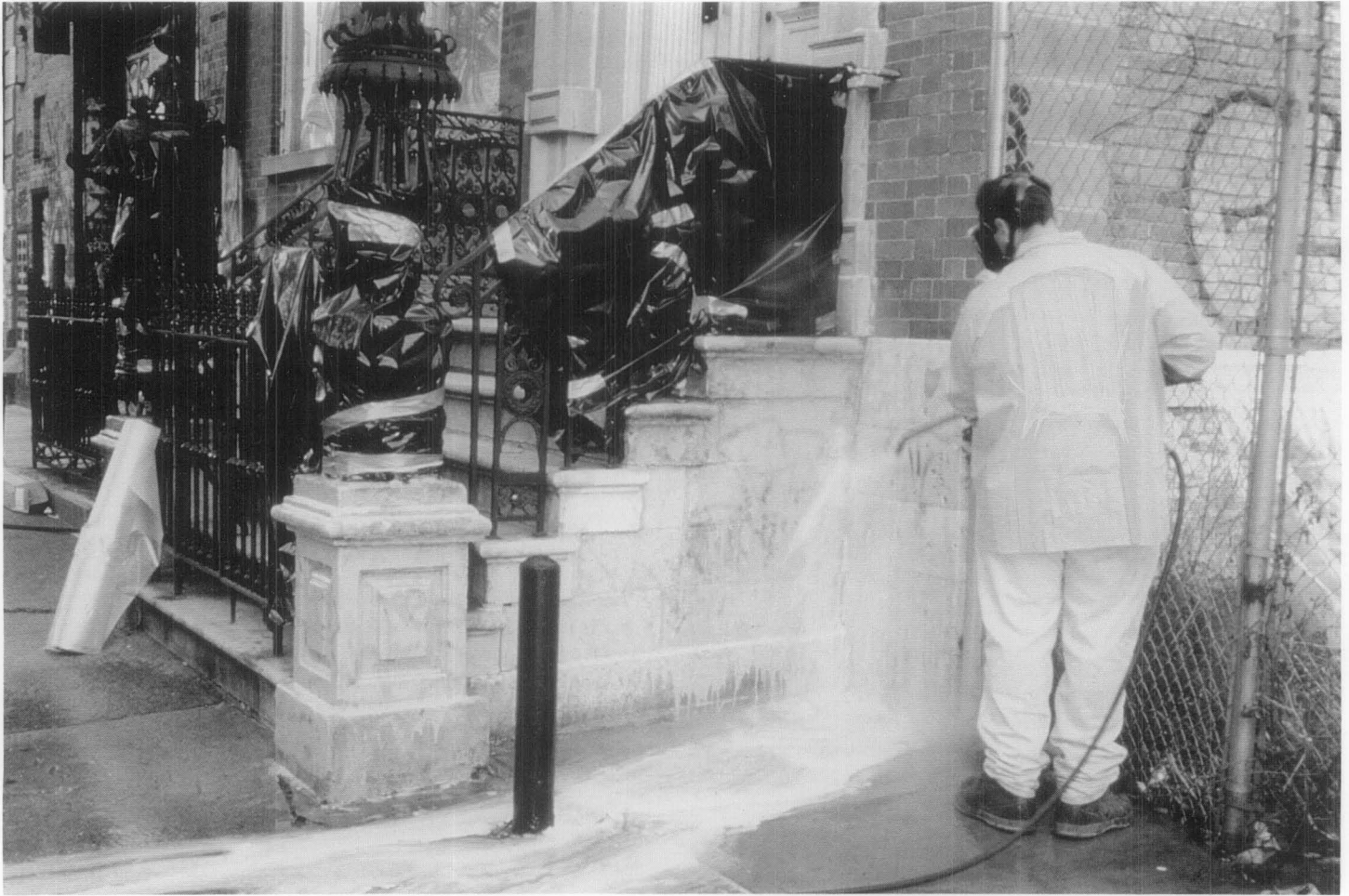
Figure 8. The cast-iron railing and light fixtures on this stone stoop have been wrapped with plastic sheeting to protect them from damage by chemicals being used to remove the graffiti. Photo: Mark A. Weber.
