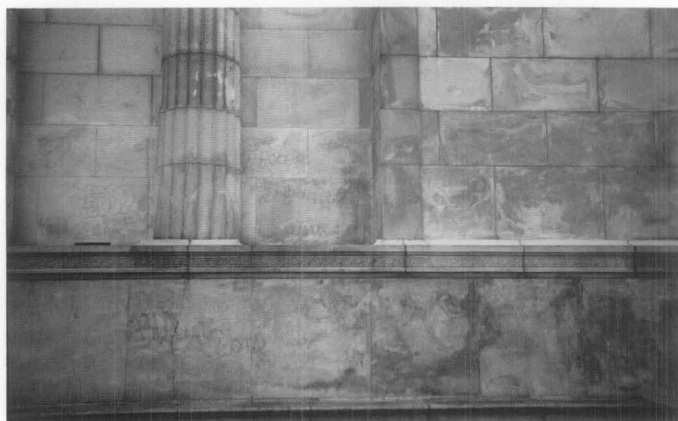
Figure 2. Harsh, but ineffective, graffiti removal methods have resulted in permanent damage to granite walls at the General Grant National Memorial in New York City. Photo: Judith M. Jacob
