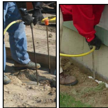
Far left: The applicator completes the interior vertical application before the flat concrete surface is poured.
