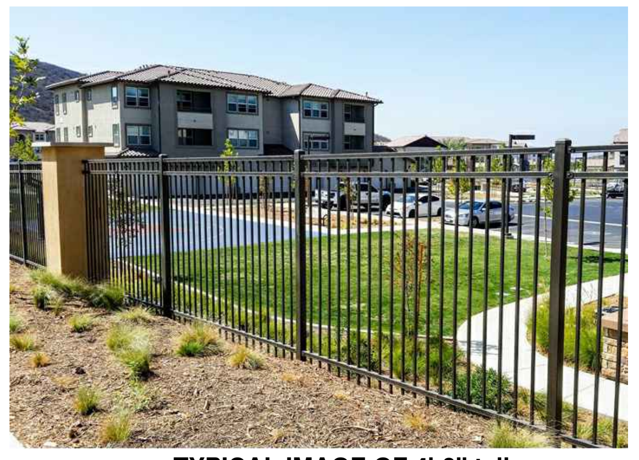
B TYPICAL IMAGE OF 4'-0" tall ALUM. FENCE - DOG PARK NO SCALE
