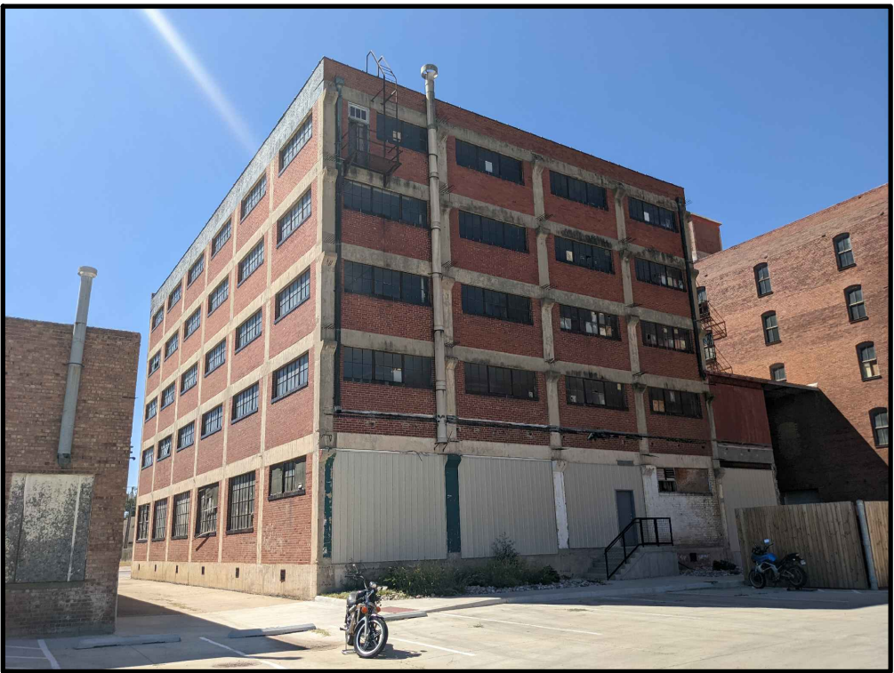
EXISTING - EAST FACADE
