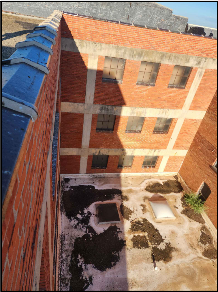
EXISTING - EAST FACADE
