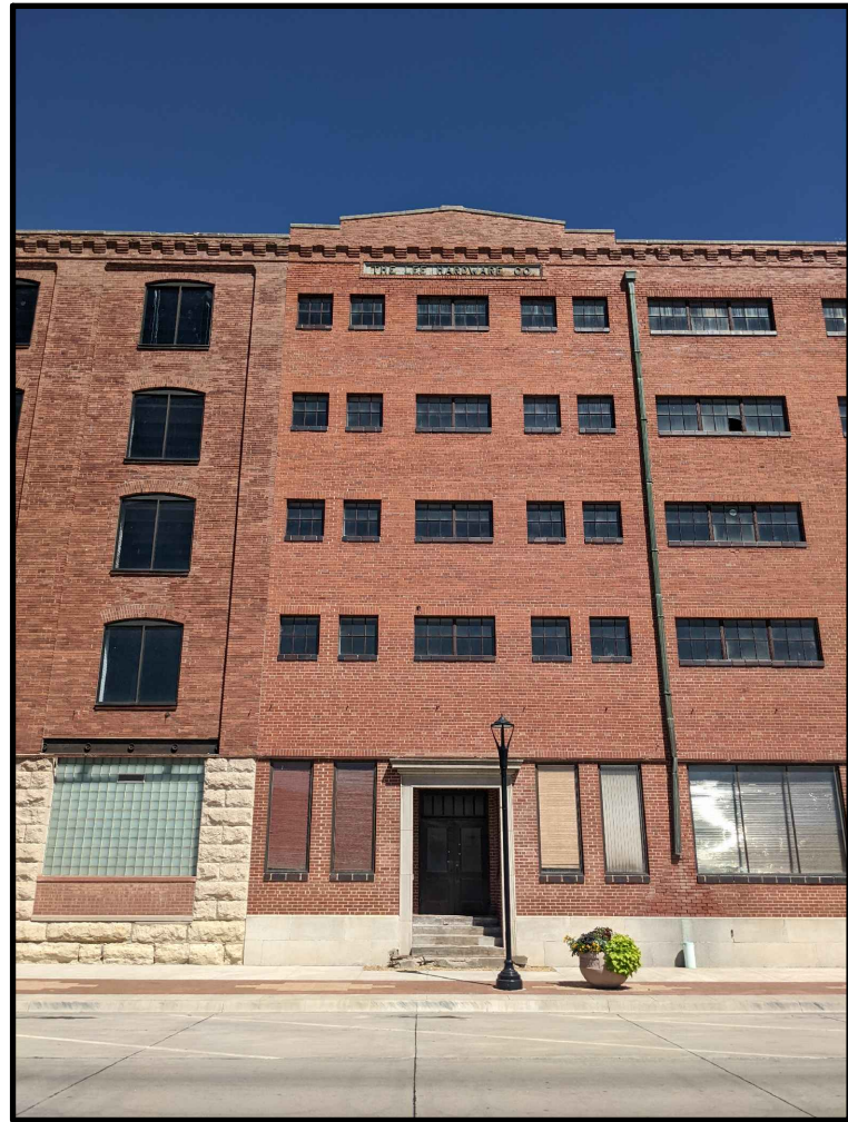
EXISTING - WEST FACADE
