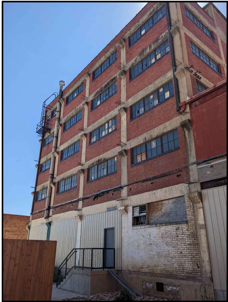
EXISTING - EAST FACADE
