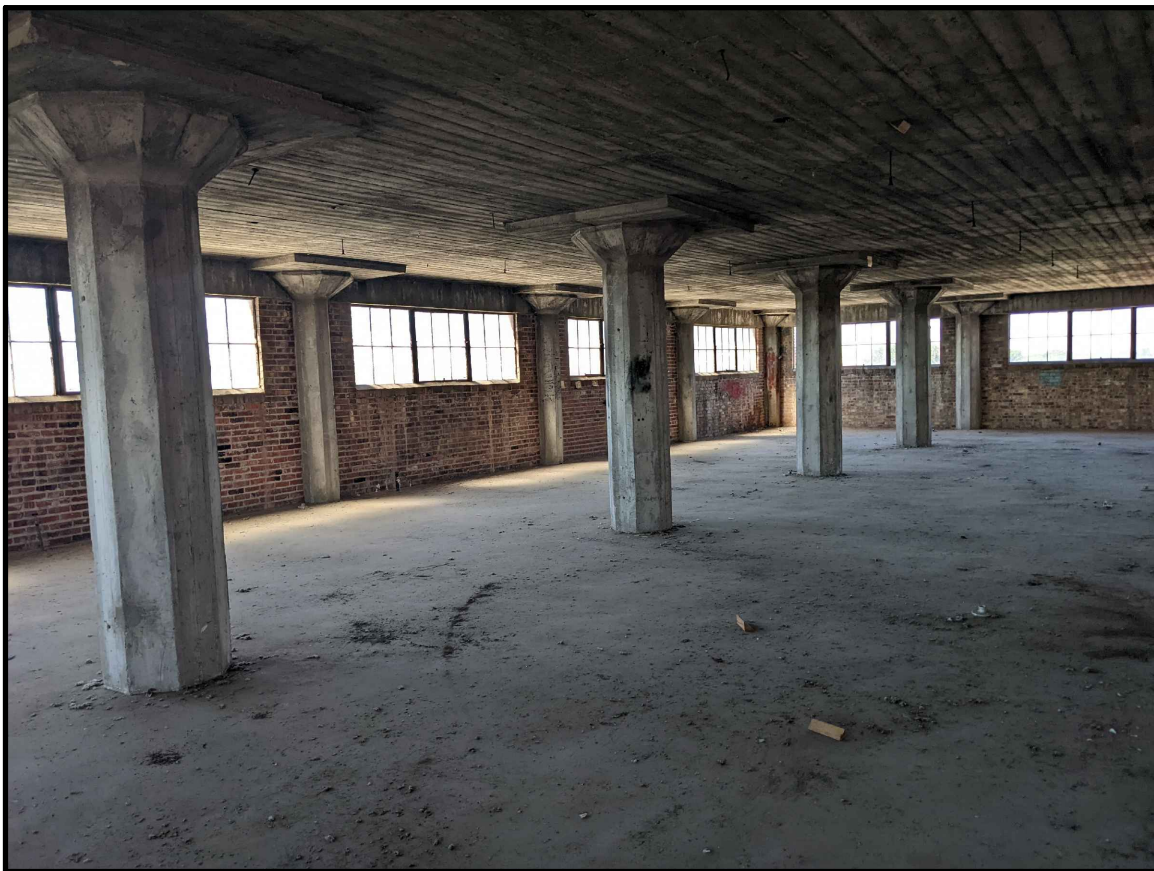
5TH FLOOR – EXISTING PHOTO EXISTING BRICK WALLS – EXPOSED, NO EXISTING PAINT: REPAIR, TUCKPOINT AS NEEDED AND CLEAN. TO REMAIN AS EXPOSED BRICK/CMU. EXISTING EXPOSED CONCRETE COLUMNS, BEAMS AND CEILING (DECK). REPAIR & PATCH AS REQUIRED. CLEAN. TO REMAIN UN–PAINTED, EXPOSED.
