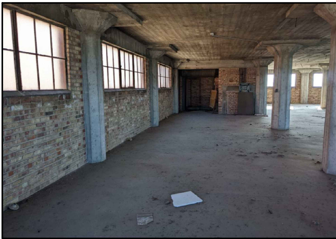
4TH FLOOR – EXISTING PHOTO EXISTING BRICK WALLS – EXPOSED, NO EXISTING PAINT: REPAIR, TUCKPOINT AS NEEDED AND CLEAN. TO REMAIN AS EXPOSED BRICK/CMU. EXISTING EXPOSED CONCRETE COLUMNS, BEAMS AND CEILING (DECK). REPAIR & PATCH AS REQUIRED. CLEAN. TO REMAIN UN–PAINTED, EXPOSED.
