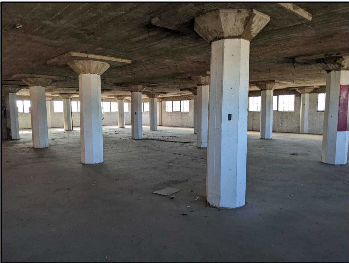
3RD FLOOR – EXISTING PHOTO EXISTING BRICK WALLS – PAINTED: REPAIR, REPLACE AND TUCKPOINT DAMAGED AREAS. REMOVE LOOSE PAINT AND DEBRIS. CLEAN AND PREP FOR NEW PAINT. EXISTING PAINTED COLUMNS. REMOVE LOOSE PAINT AND DEBRIS. REPAIR DAMAGED AREAS. PREP FOR NEW PAINT. EXISTING EXPOSED CONCRETE BEAMS, COLUMN CAPS AND CEILING (DECK). REPAIR & PATCH AS REQUIRED. CLEAN. TO REMAIN UN–PAINTED, EXPOSED.
