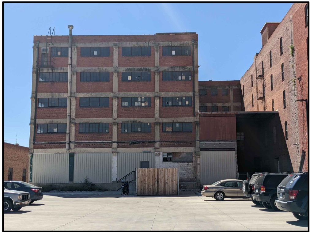
EXISTING - EAST FACADE
