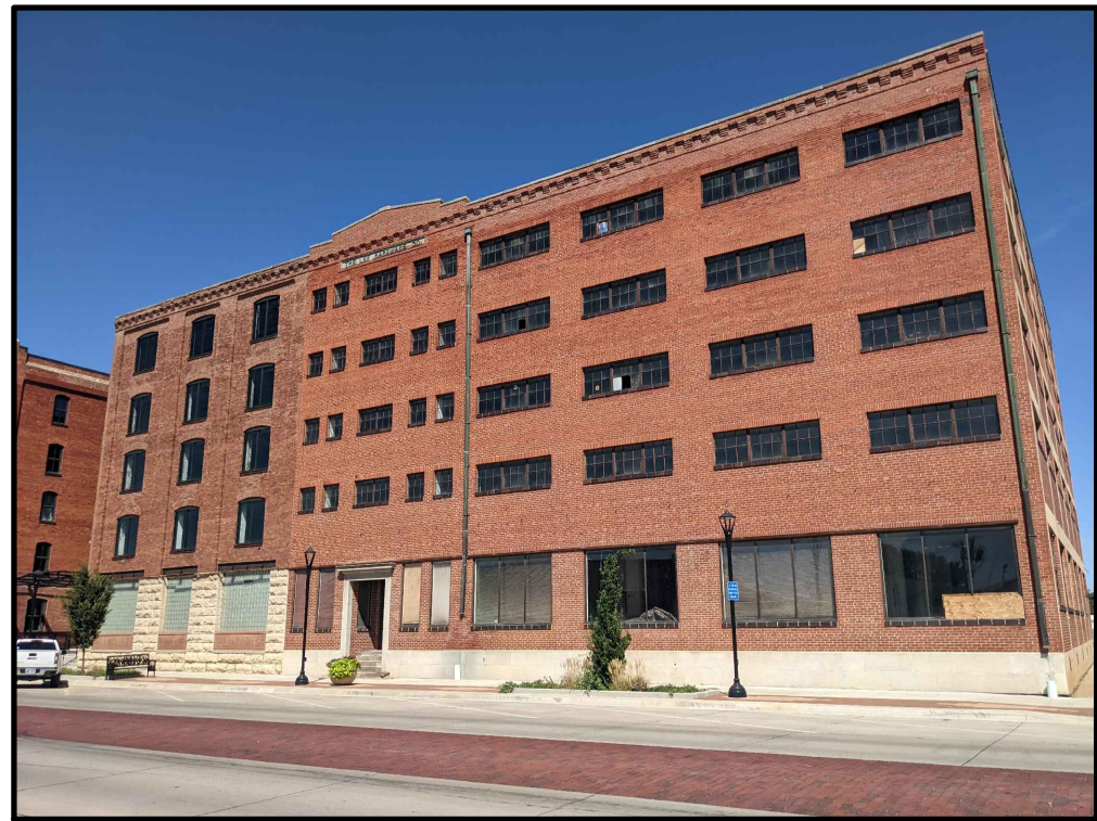
EXISTING - WEST FACADE
