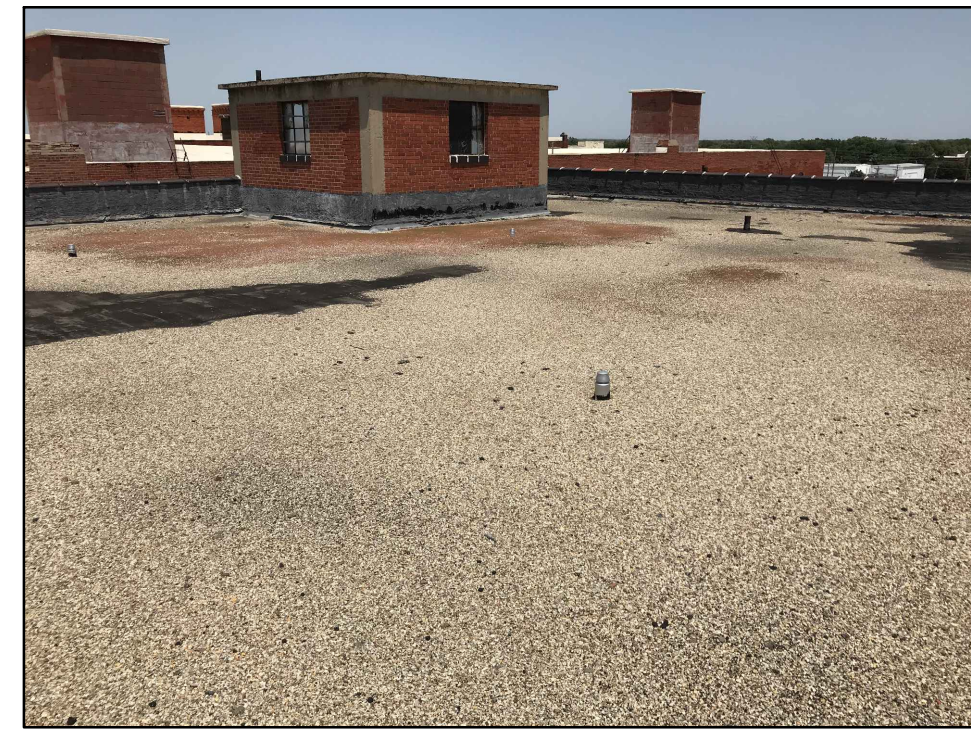
B EXISTING ROOF PHOTOS
