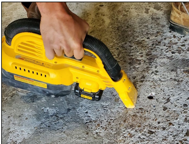
Image 3 – Clear and sweep/vacuum sample area
