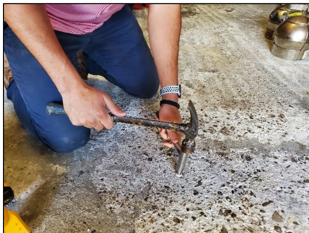
Image 5 – Installation of vapor pin
