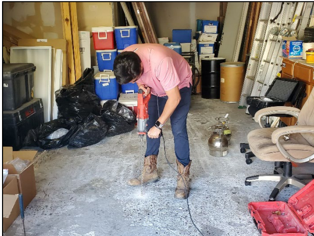
Image 1 – Initial drilling activities
