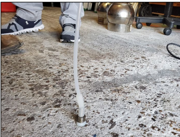
Image 6 – Connection of tubing to vapor pin
