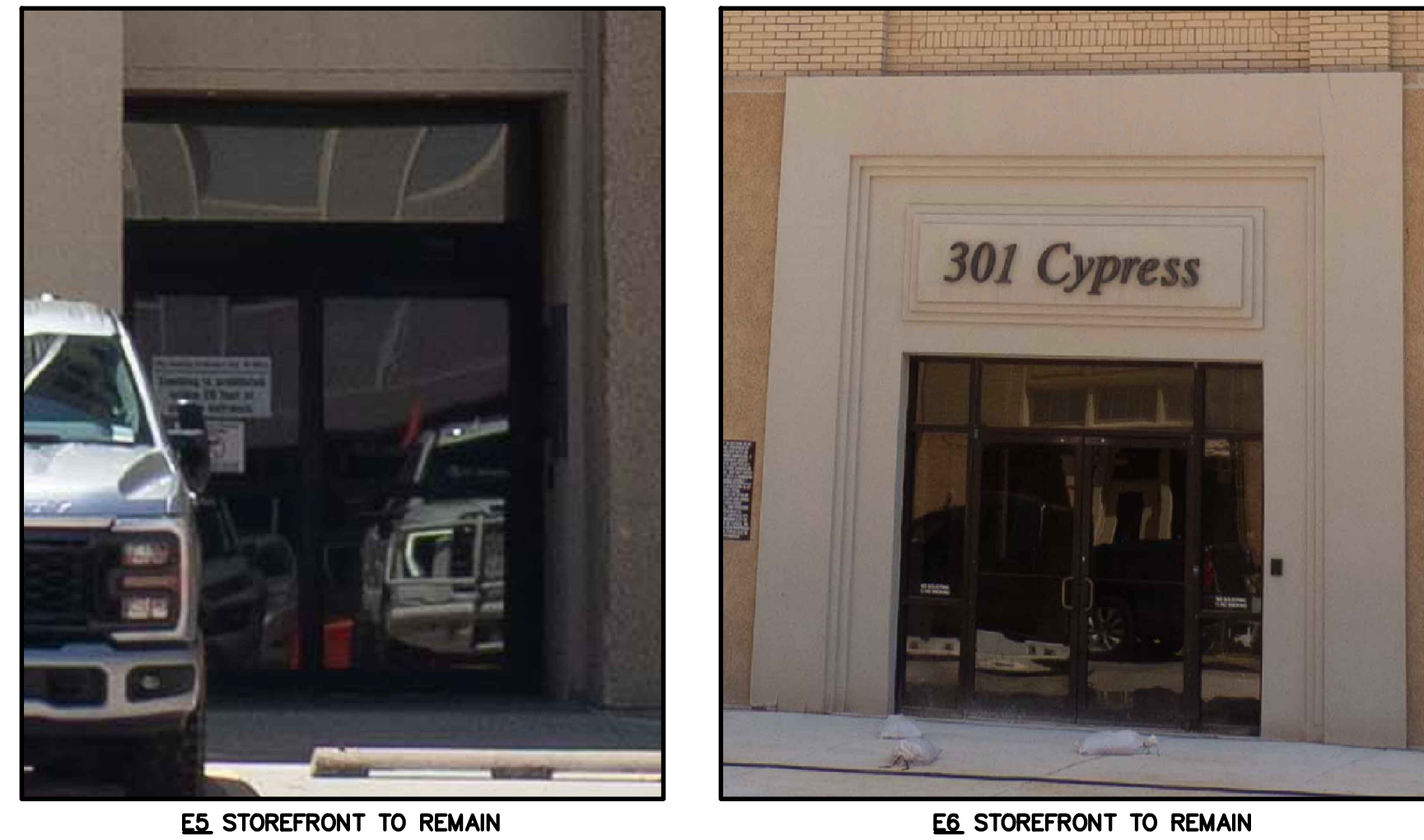
C PHOTOS: EXISTING WINDOWS
