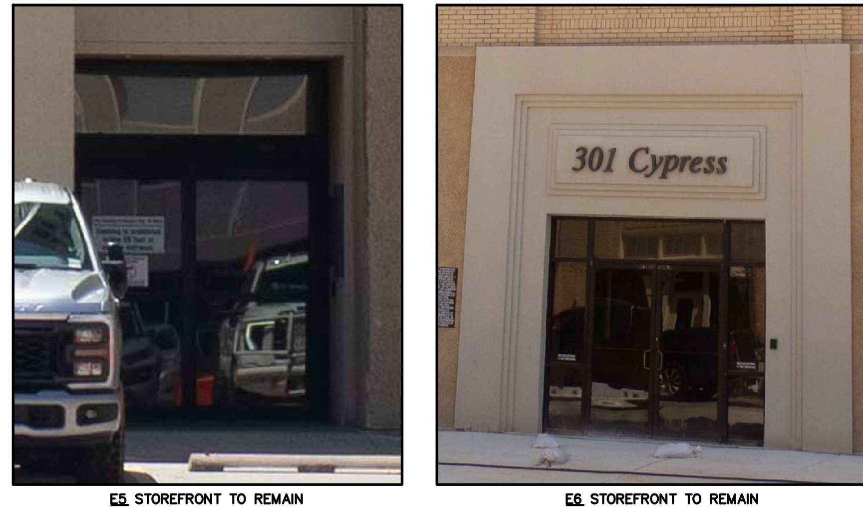
C PHOTOS: EXISTING WINDOWS
