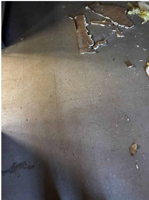
1. 12"x12" floor tile with black mastic current samples 1-3
