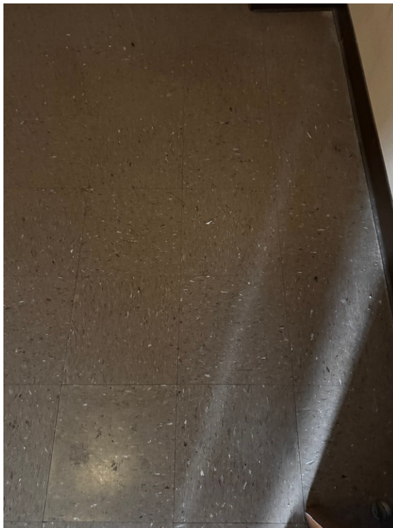
2. Former identified floor tile ACM samples (068-070)
