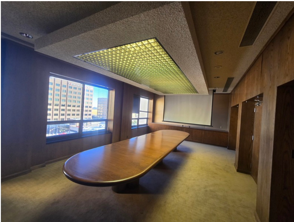
5. HA-2 ceiling material in 7th floor board room samples 4-6
