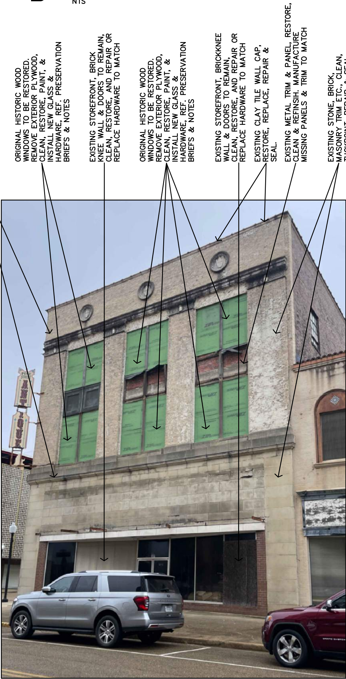
A SEARS BUILDING EXISTING EAST PHOTO NTS
