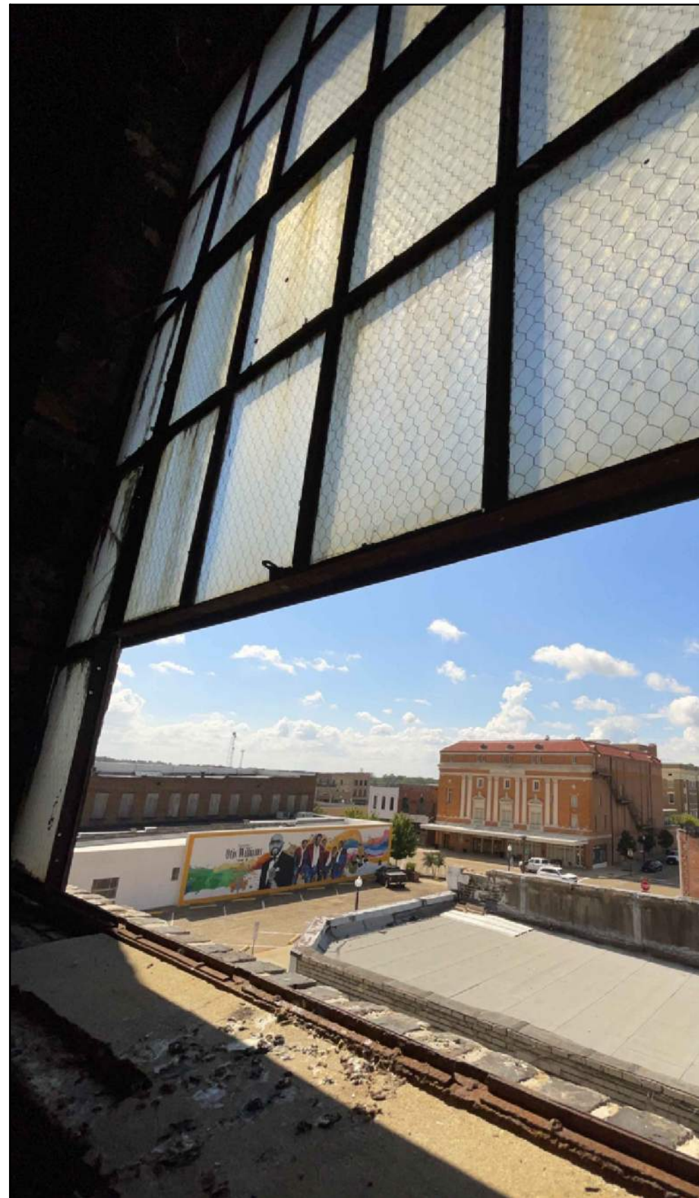
C SEARS BUILDING EXISTING STEEL WINDOWS
