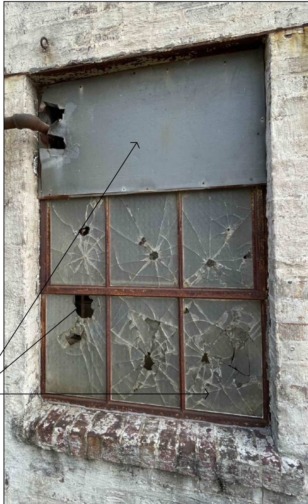
D SEARS BUILDING EXIST'G STEEL WINDOWS
