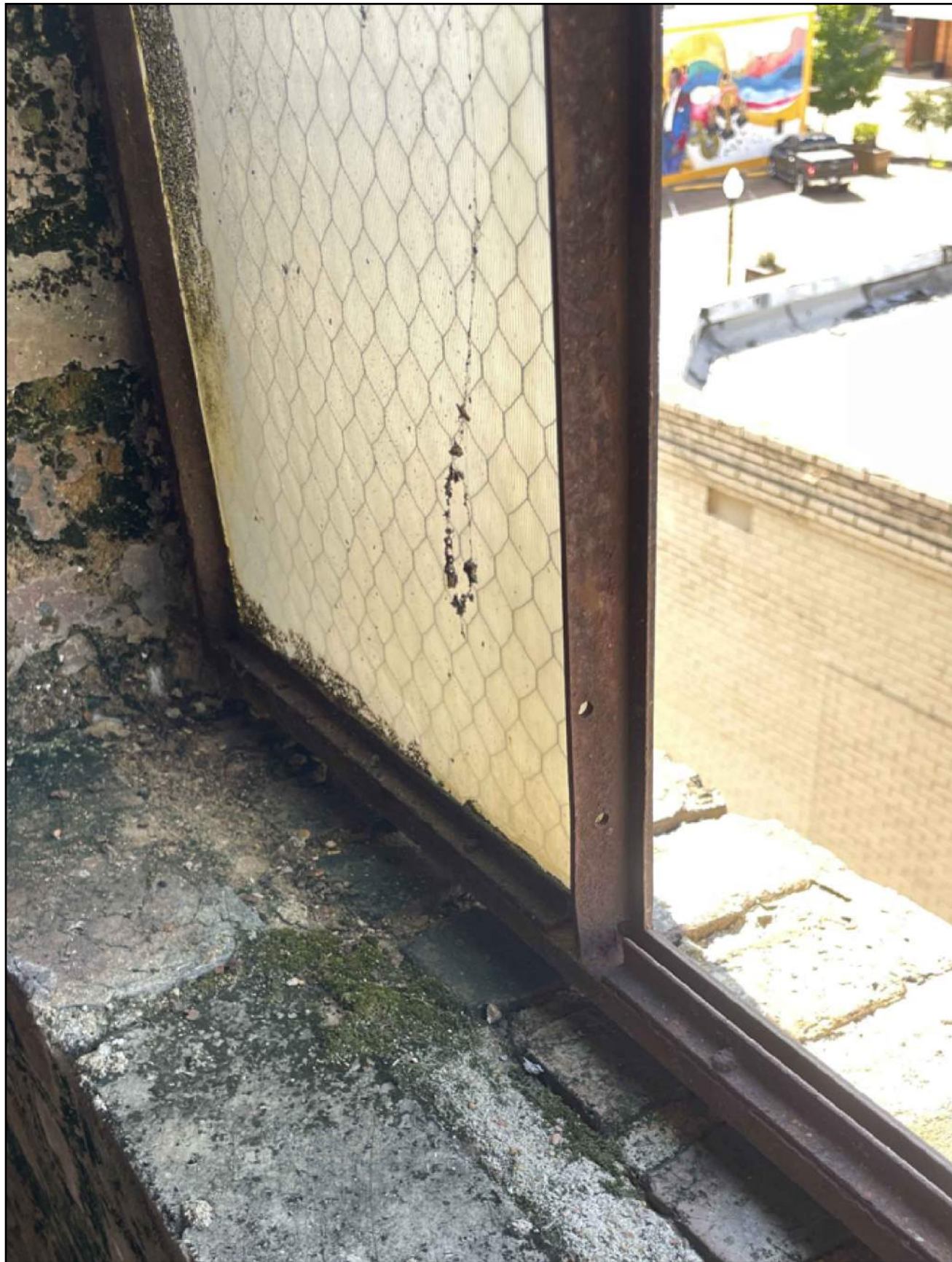
F SEARS BUILDING EXIST'G STEEL WINDOWS
