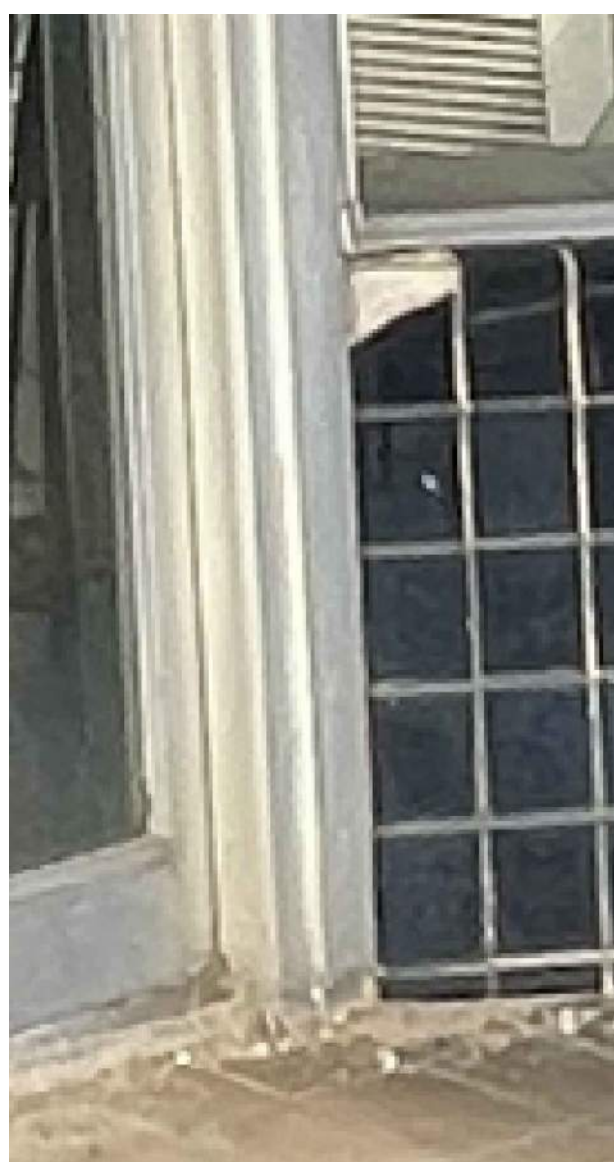
C GAZETTE BUILDING EXISTING PHOTOS PINE 305 3"=1'-0"
