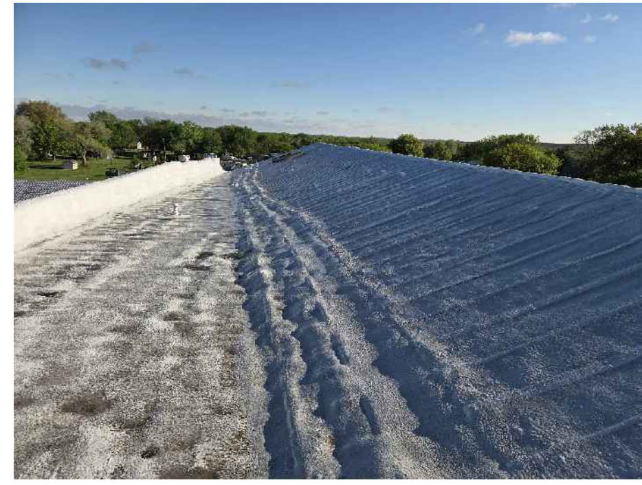
X PHOTOGRAPH VIEW OF WEST ROOF AREA LOOKING NORTH
