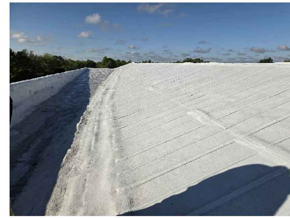
AA PHOTOGRAPH VIEW OF EAST ROOF AREA LOOKING SOUTH
