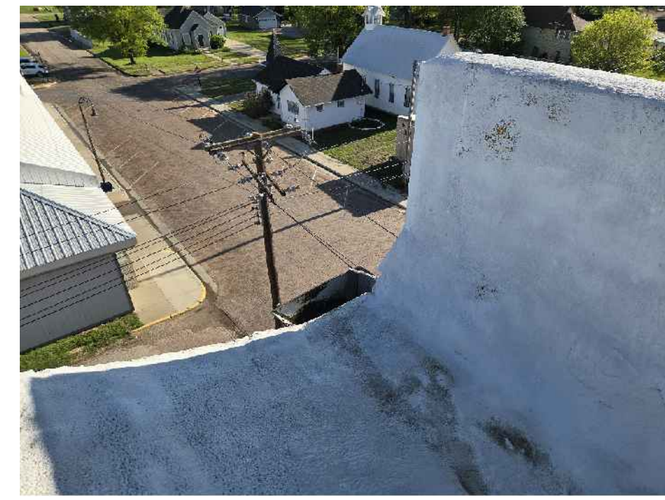
Z PHOTOGRAPH VIEW OF N.E. ROOF AREA LOOKING NORTH
