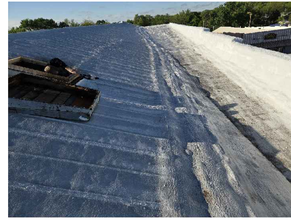
W PHOTOGRAPH VIEW OF WEST ROOF AREA LOOKING SOUTH
