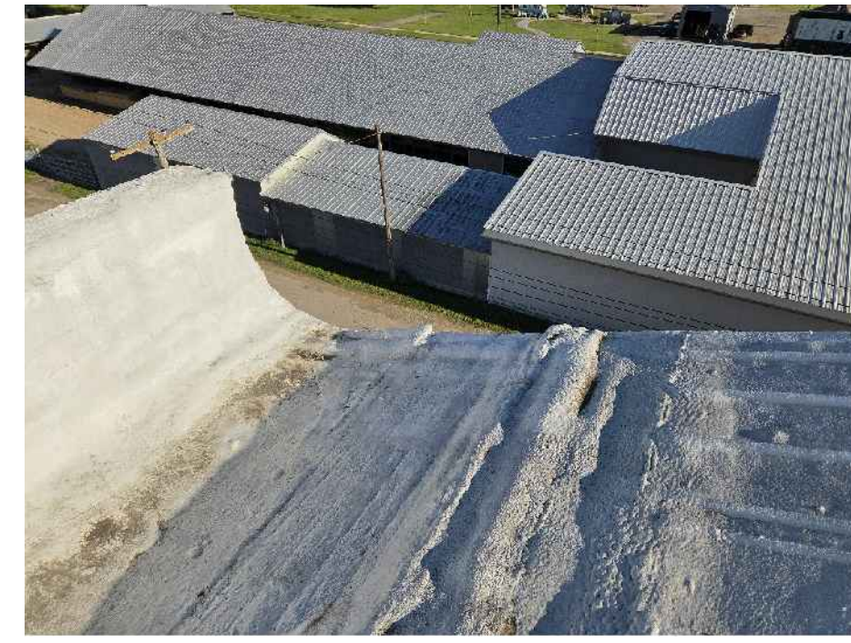
V PHOTOGRAPH VIEW OF N.W. ROOF AREA LOOKING NORTH
