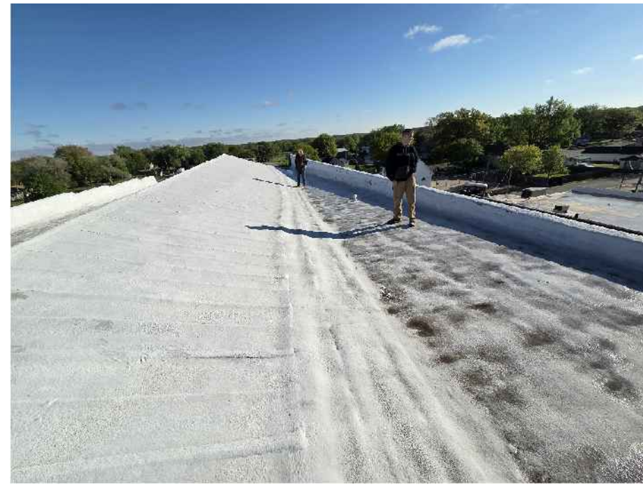
Y PHOTOGRAPH VIEW OF EAST ROOF AREA LOOKING NORTH
